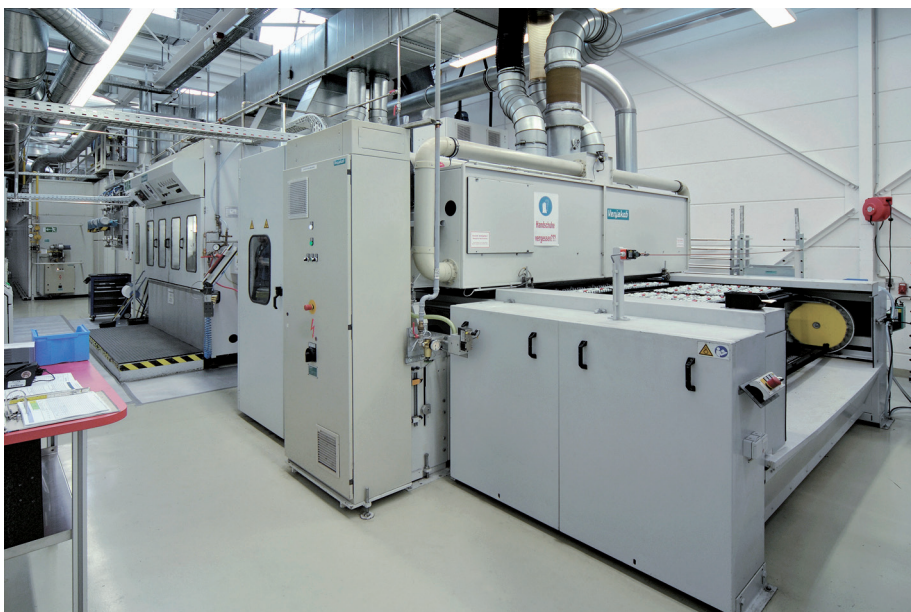
Fig. 2: The Openair plasma system (3rd unit from the front) takes up only one metre of a painting line with an overall length of 25m (Photo Plasmatrete)
